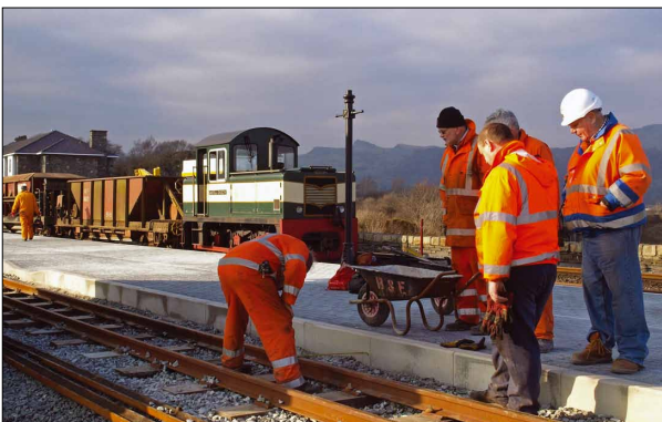
The volunteers check the critical measurement between the platform edge and the running rail. Stuart McNair (R) observes.
