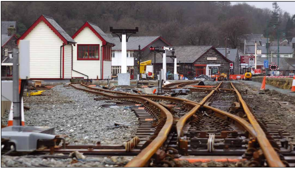
Caernarfon straight on; Harbour Station, turn left! The track layout installed and awaiting tamping. Note the point motor, left.
