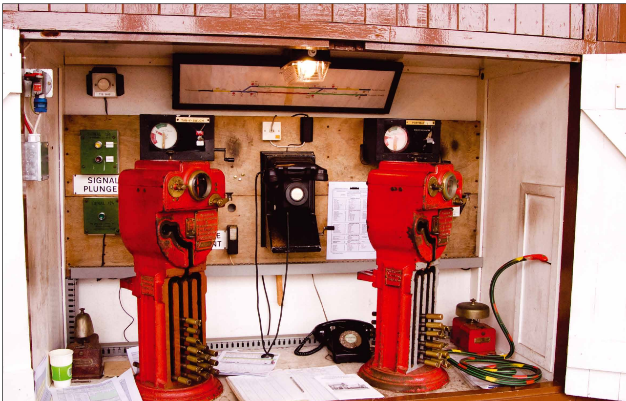
Conventional ETB has run the Ffestiniog Railway safely for years. It may be obsolescent, but it can be maintained by the FfR, it has high utility and good reliability. Extras added include remote operator working, starting signal clearance, and automatic operation of points. It was considered desirable not to have another railway (the WHR) with a different system, as staff work on both - hence the development work and the clever solution.
